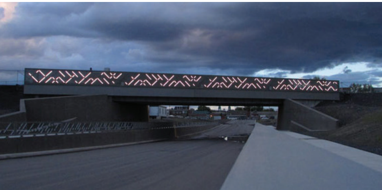
Pont ferroviaire, campus Outremont © Civiliti
